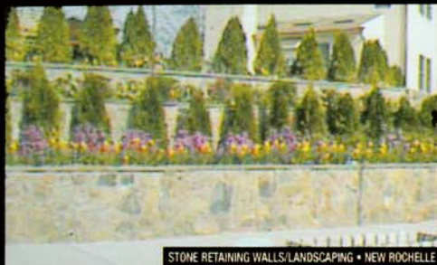
STONE RETAINING WALLS/LANDSCAPING • NEW ROCHELLE
