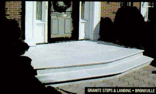
GRANITE STEPS & LANDING • BRONXVILLE
