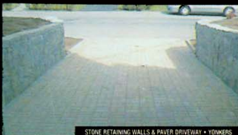
STONE RETAINING WALLS & PAVER DRIVEWAY • YONKERS
